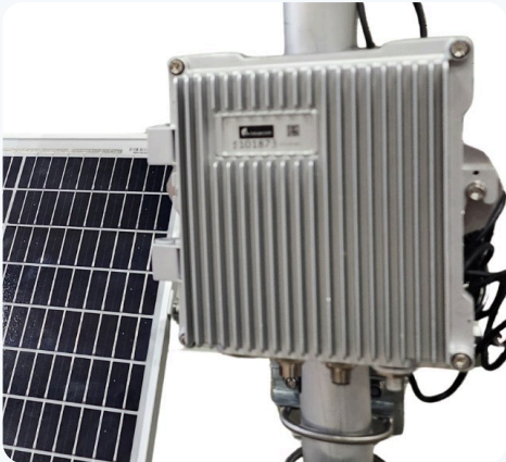
SynaptiX Collector and solar Data acquisition, telemetry and solar charging
